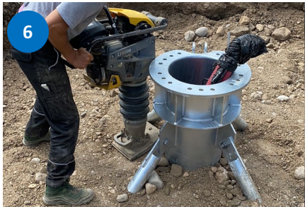
6 Bring in the excavated material and compact in layers
