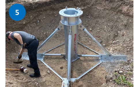
5 Lifting into the hole with the excavator and arrange
